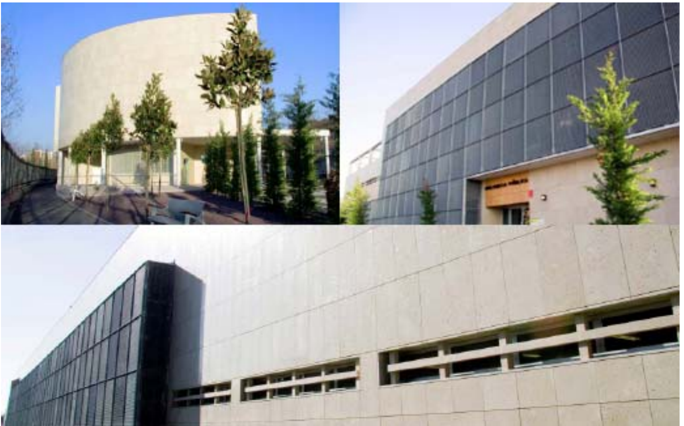
State Public Library of Ciudad Real, Spain, inaugurated on 22 nd December 2010
